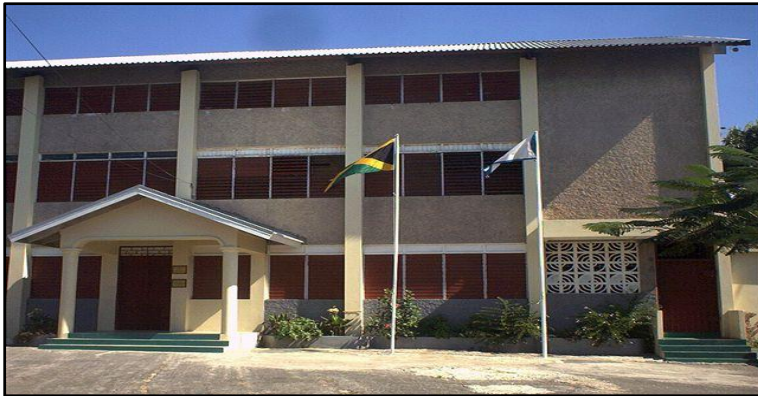
Food Preparation/Electrical Installation/Remedial Campus
