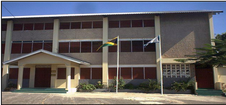
Food Preparation/Electrical Installation/Remedial Campus
